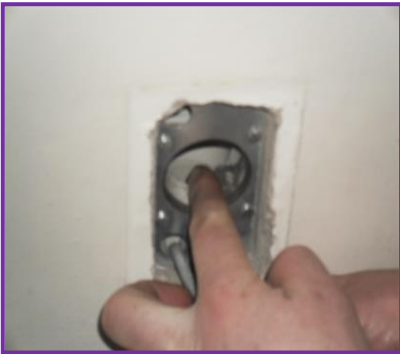
4. Clean around the wall port
