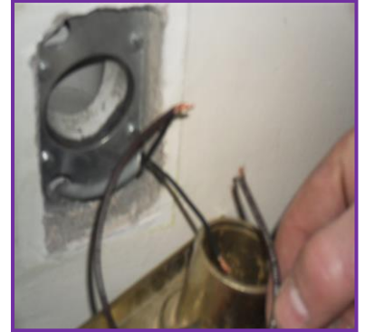
3. Remove old inlet from the wall, Disconnect Low Volt Wires
