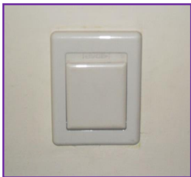
7. Plumb inlet, tighten screws and fit inlet trim, making sure the larger part of trim is facing upwards
