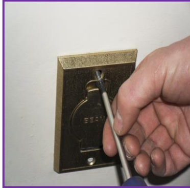
2. Unscrew old inlet from wall
