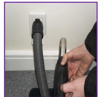
9. Test the inlet is working correctly and ensure no leaks
